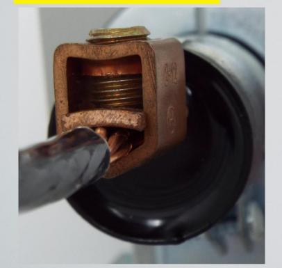
Caution: Failure to properly connect the wire can cause the connection to overheat and possibly rupture the tube
